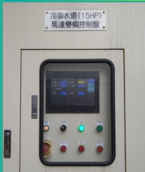
Installation of variable frequency control system for cooling tower fans
